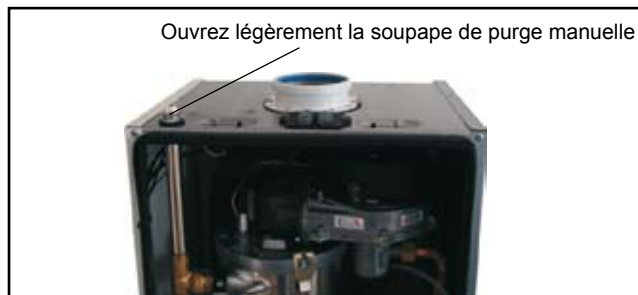
Illustration: soupape de purge manuelle
